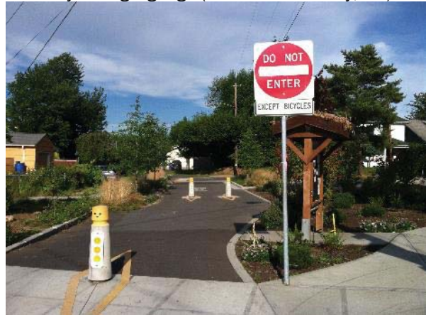
Path connection for walking and biking created as part of a street vehicle closure (Portland, OR)
